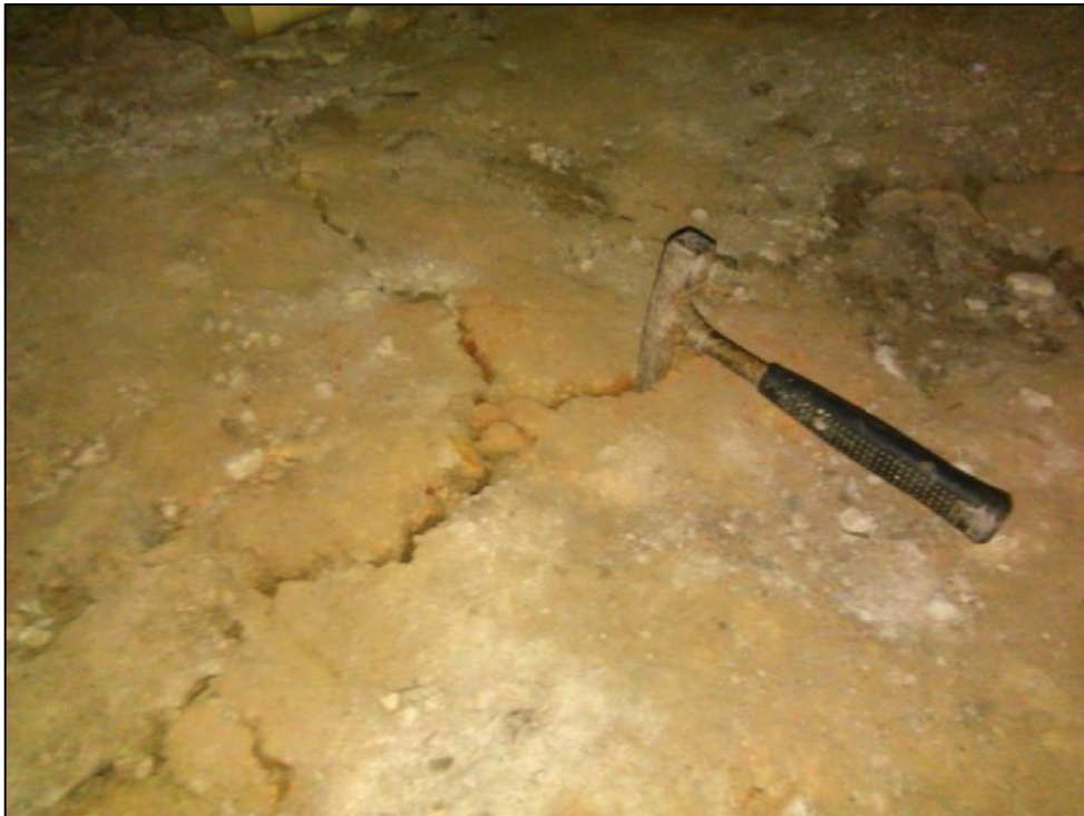
Figure 7: Facing north beneath building near Bore 8 (Observation 1) showing soil cracking
