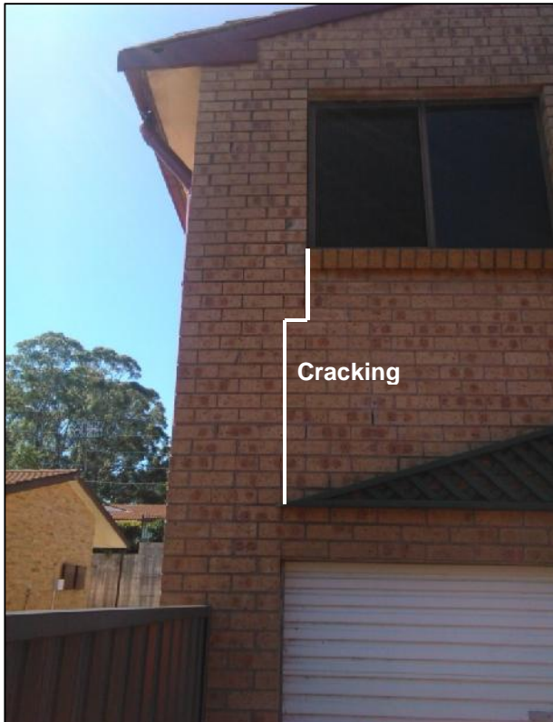
Figure 6: Facing north from near Bore 8, showing cracking in existing building beneath window edge
